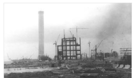
Drax Power Station during construction
